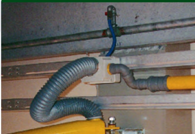
90SCATD010 Derivation box for cables and tubes for articulated arm
